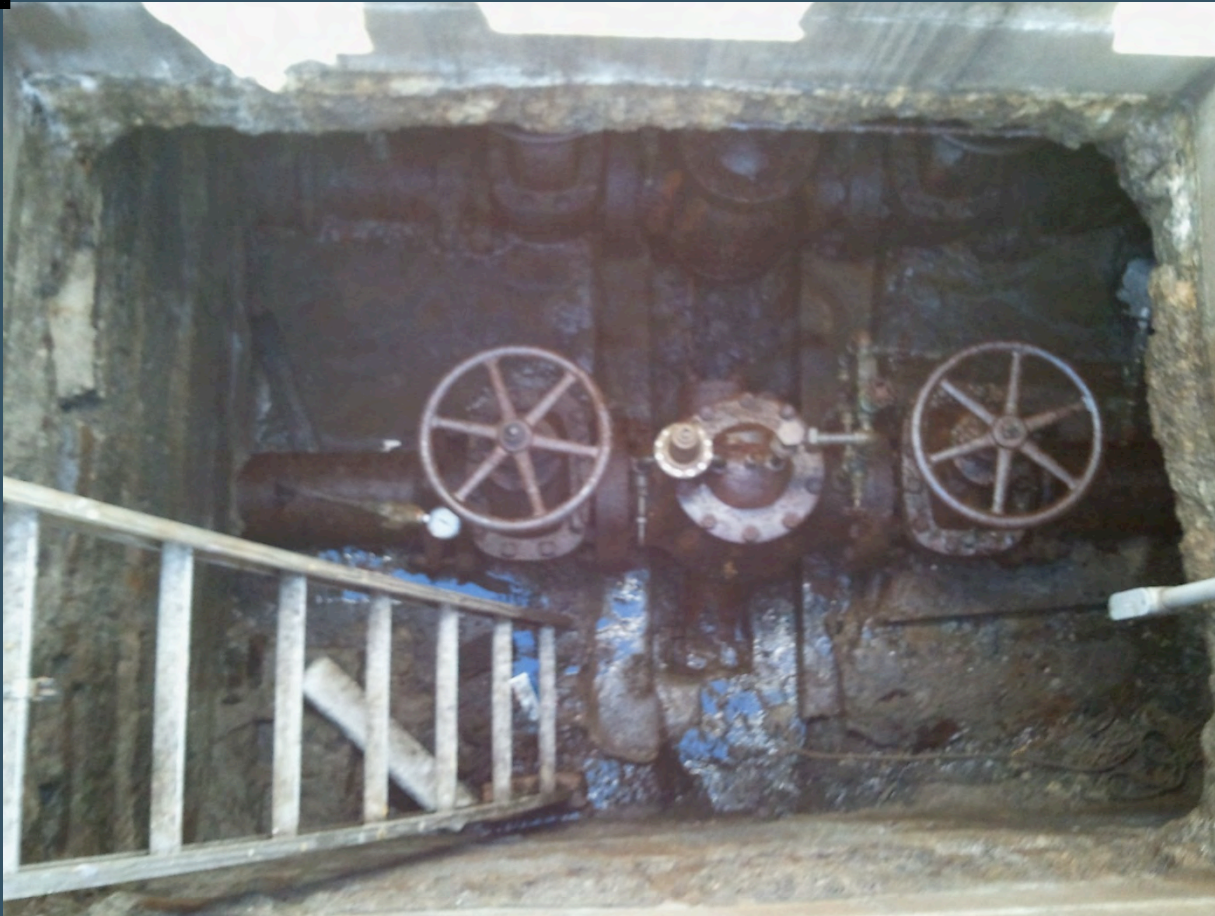
Current Nelson Street Vault, March, 2011
