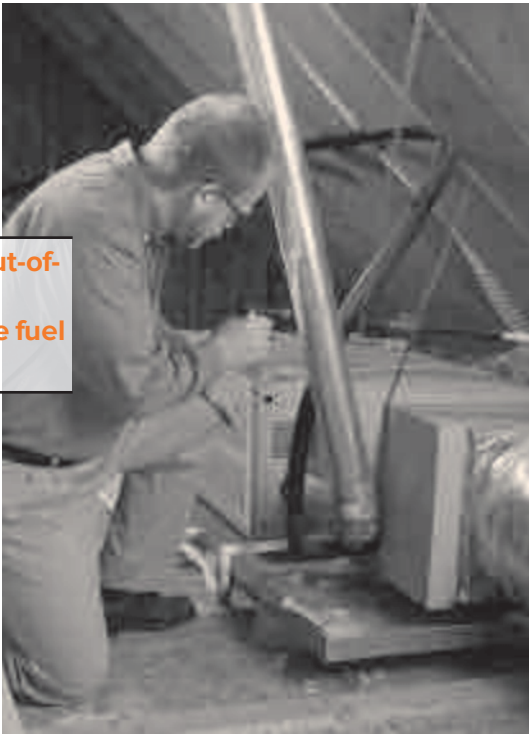
An energy upgrade technician inspects the furnace and measures the efficiency and performance of a residential heating system.
