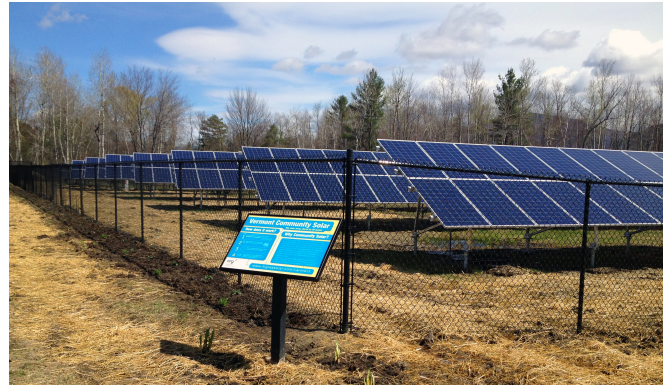
Rutland Vermont Community Solar Project (Photo: Business Wire)
