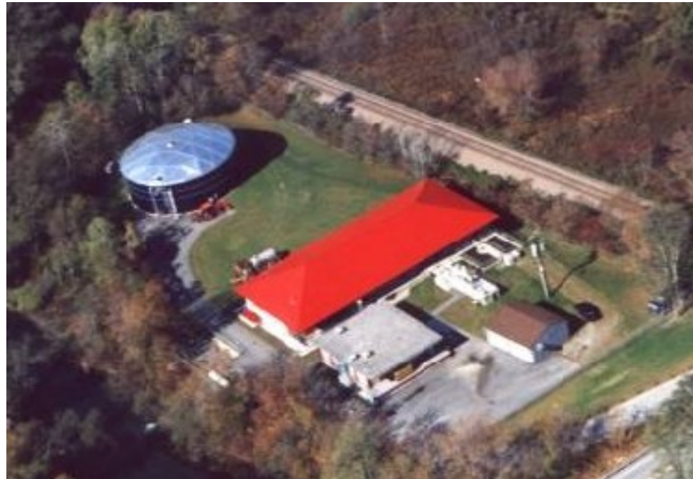
Castleton Wastewater Treatment Facility
