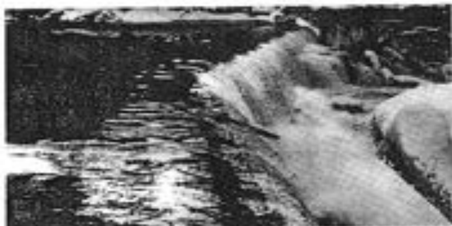
Part of four miles of water spilling over falls at lower Salsburg Intermediate School
